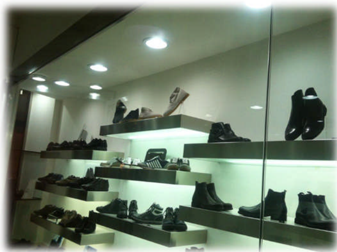
Place: Boutique Caserta Led lamp type: Down light led 30W white. Interior shop window.
